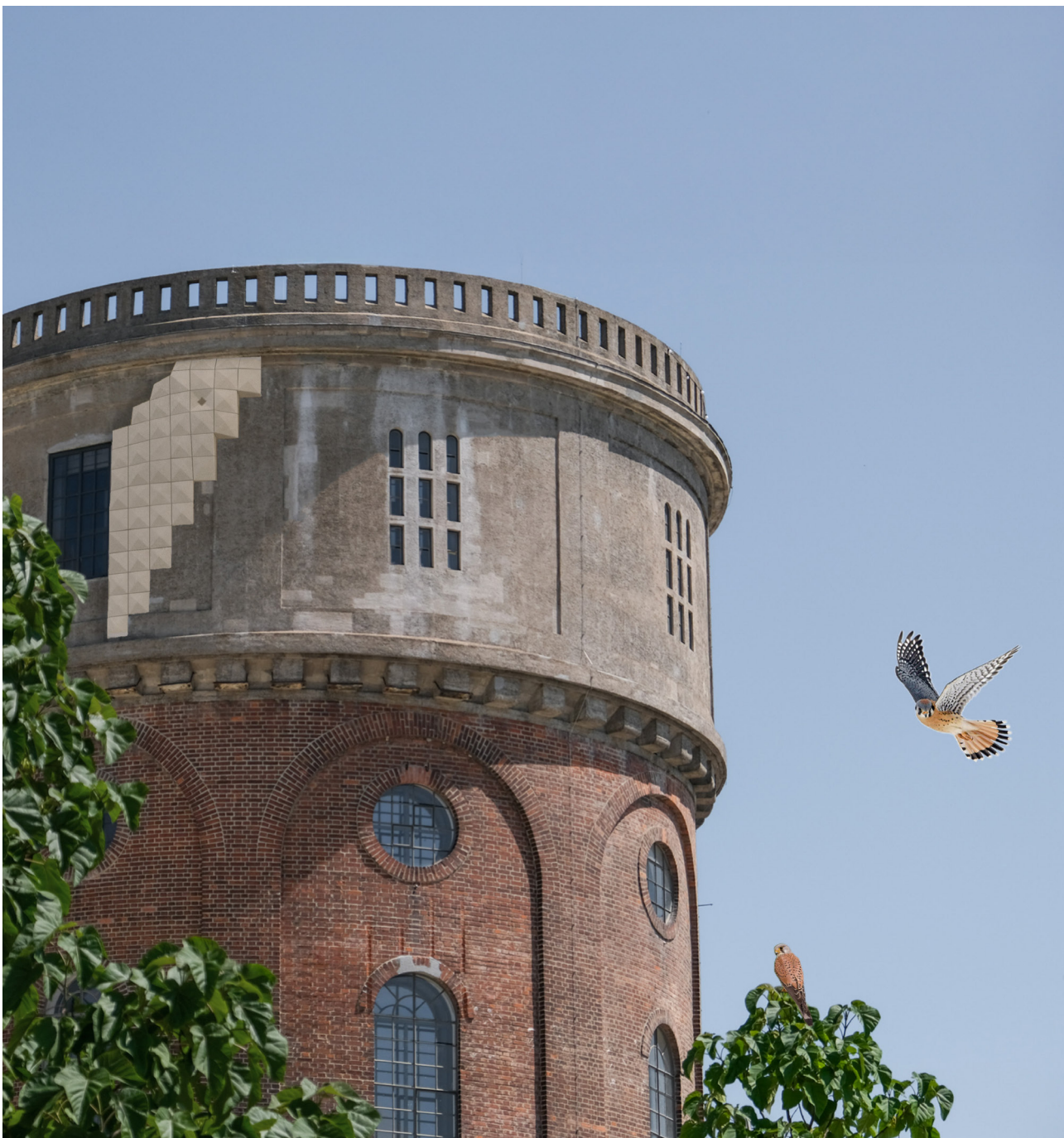
Main installation on the tower
