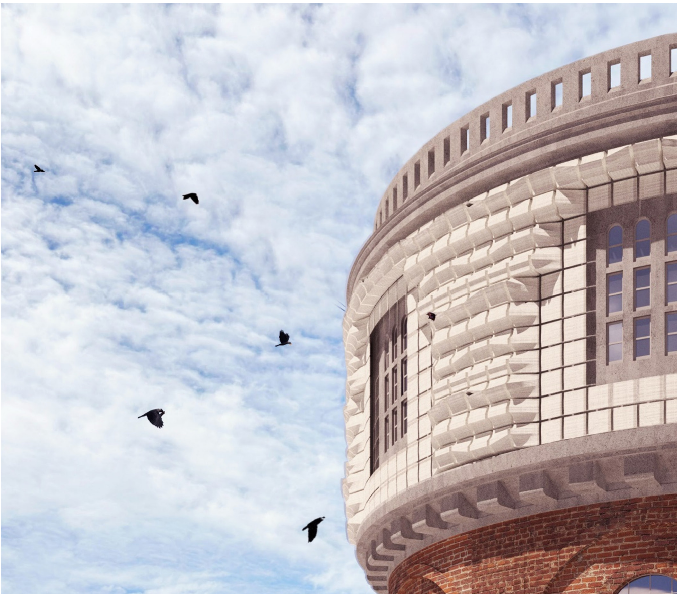
South-West View of the Tower
