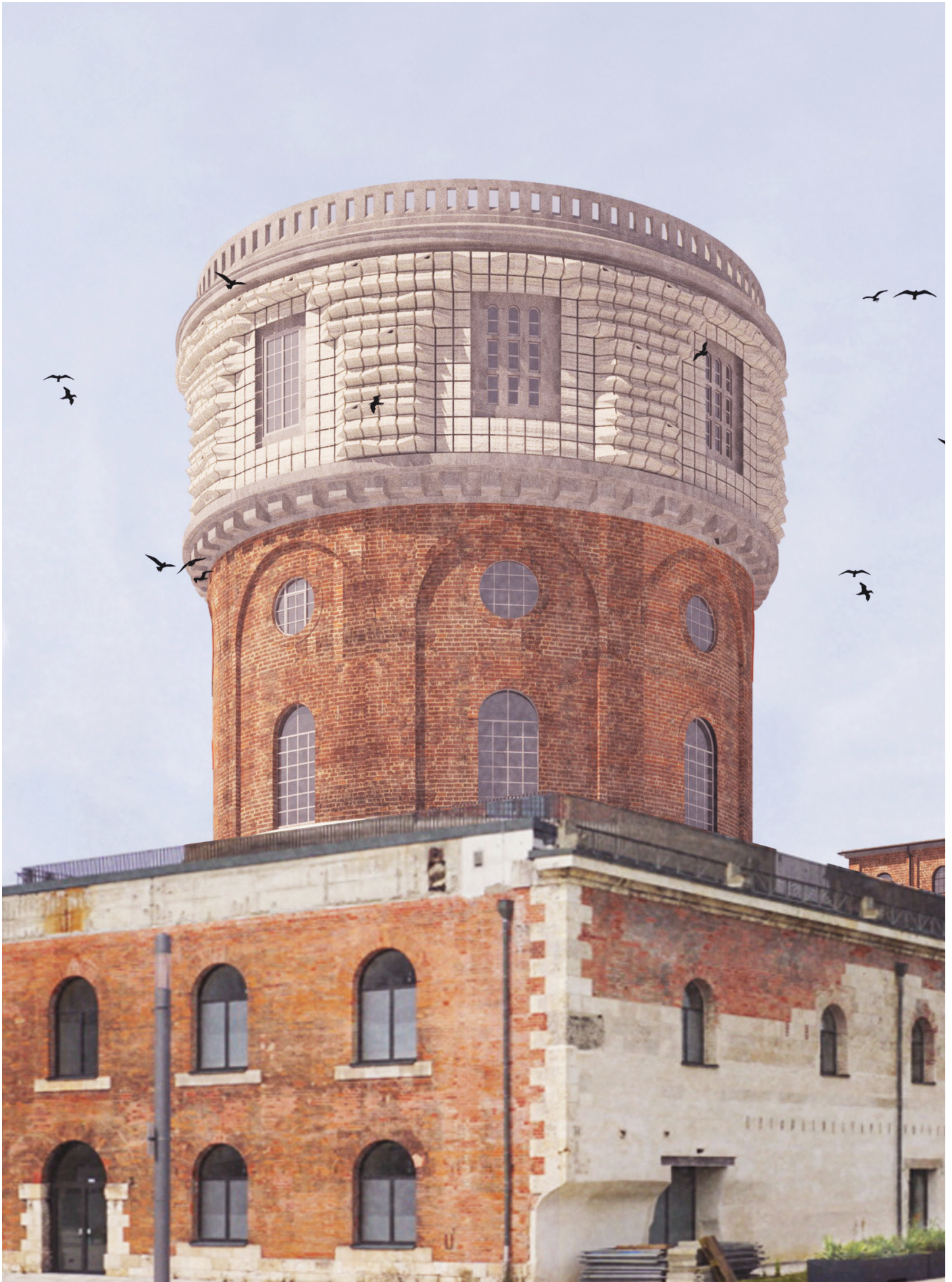
South-East View of the Tower with New Facade
